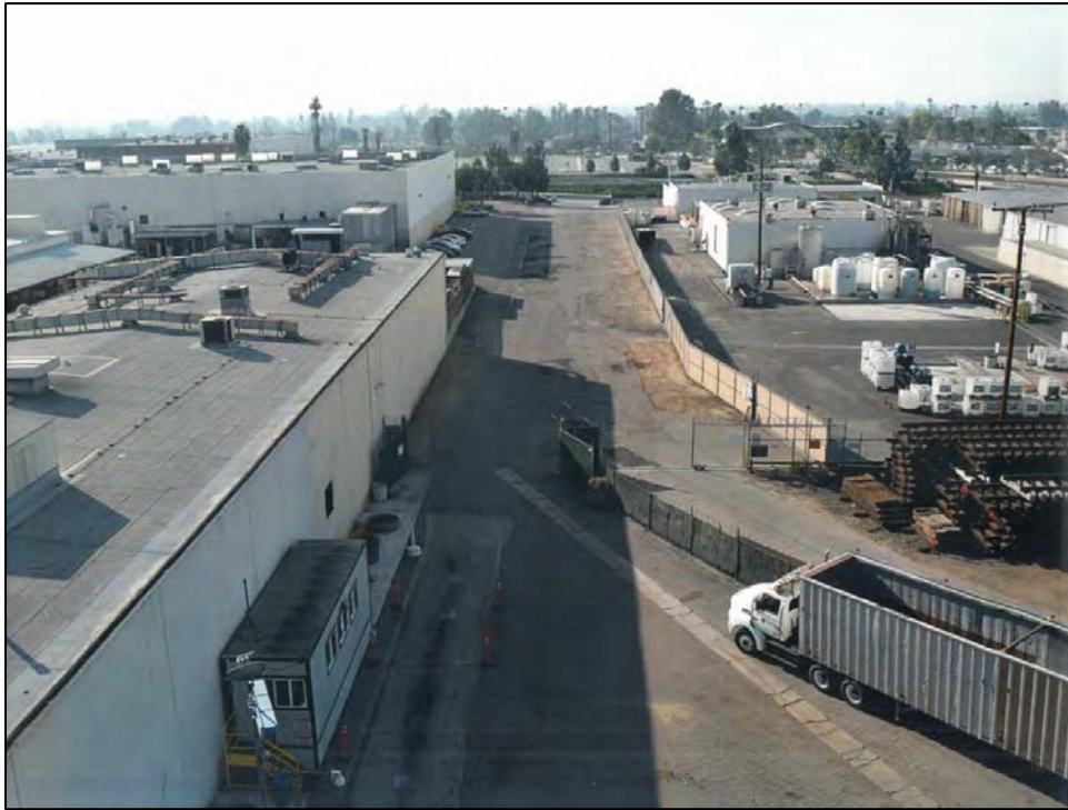
View of project site driveway, facing south
